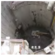
1. Seattle, USA, Beacon Hill Tunnel, pre-excavation- grouting
