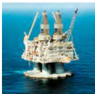
3. Lake Maracaibo, Venezuela, oil well squeeze (repair) cementing
