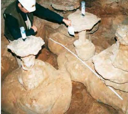
Grouting tests at the job-site
