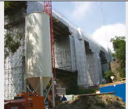
Concrete and masonry repair
