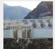
7. Muratlin, Turkey, Hydropower Station, ridge slot grouting
