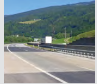
Bridge strengthening, TU Graz
