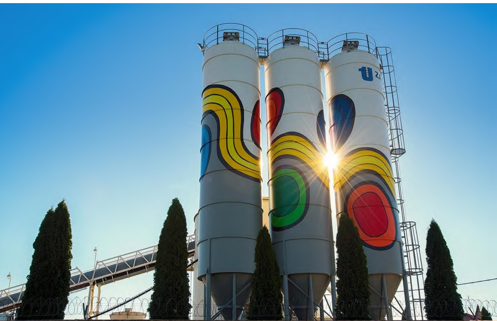
Ready mix-batch plant, Hlohovec, Slovakia
